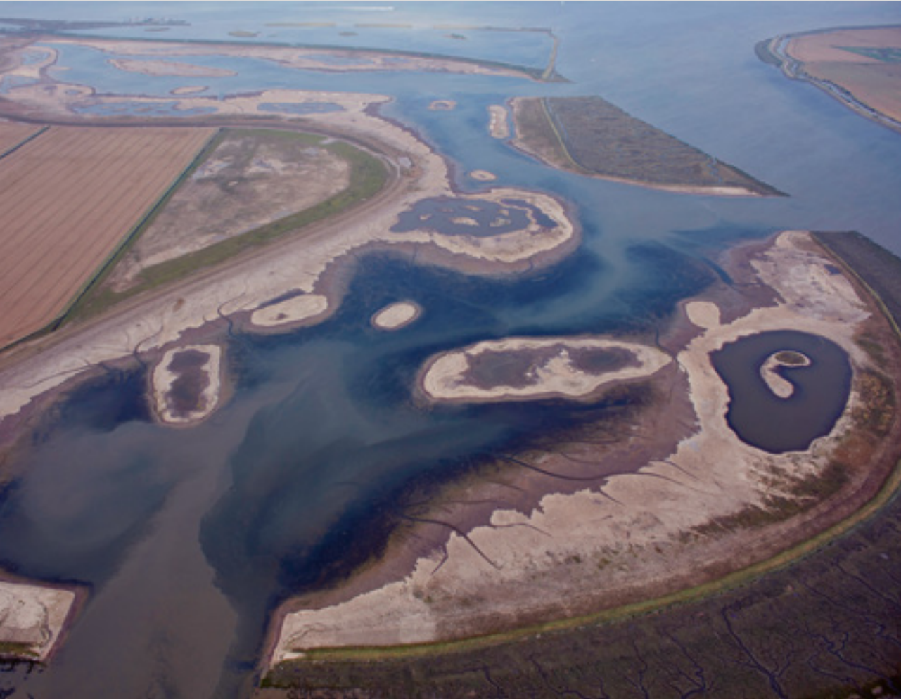
Wallasea Island Wild Coast Project: a wetland designed to provide valuable habitat for wildlife, both now and under a range of future climate conditions.
