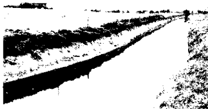
Section of River Ouzel downstream from photograph on page 5, after channel dredging and bank clearance by Water Authority in 1981. Photo: K. Taylor.
